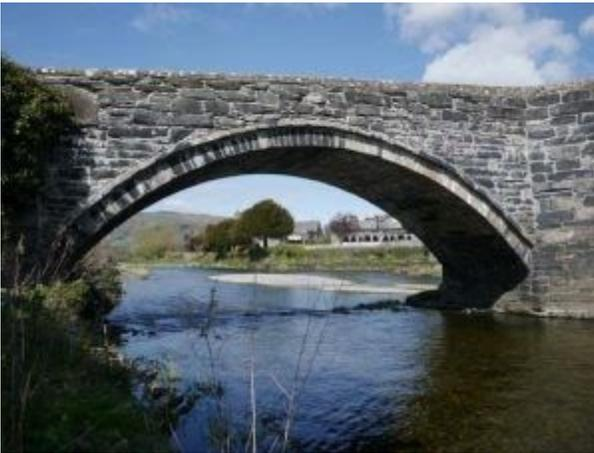
An arch bridge supports loads by distributing compression across and down the arch. The structure is always pushing in on itself.
