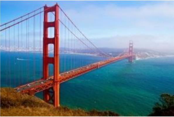
The towers (piers) of a suspension bridge are in compression and the deck hangs from cables that are in tension. The deck itself is in both tension and compression.
