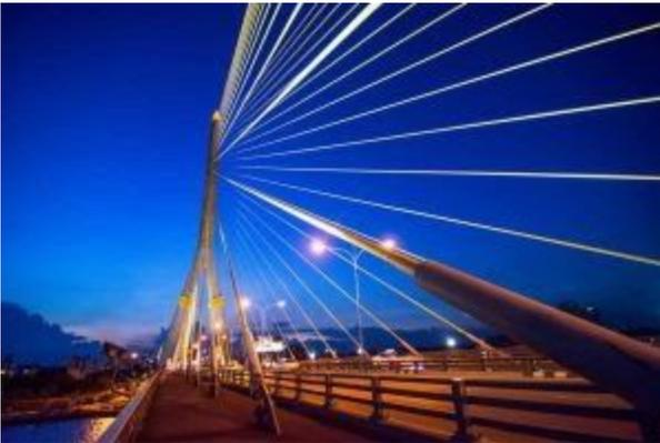
A cable-stayed bridge is similar to a suspension bridge. However, the deck hangs directly from the piers on cables. The piers are in compression and the cables are in tension. The deck experiences both forces.
