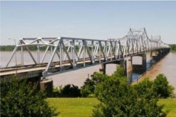
A cantilever bridge is one of the simpler forms to understand. Basically, it addresses the forces of tension (pulling) above the bridge deck and those of compression (pushing) below.
