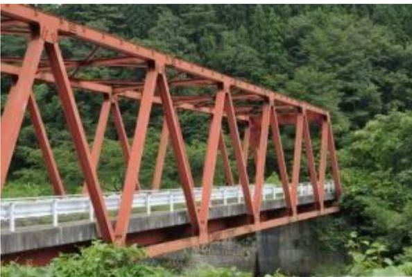
A truss bridge is a variation of a beam structure with enhanced reinforcements. The deck is in tension. The trusses handle both tension and compression, with the diagonal ones in tension and the vertical ones in compression.
