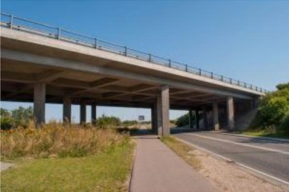
A beam bridge has its deck (beam) in tension and compression. (The beam can be squeezed and stretched depending on conditions.) The abutments are in compression, which means they are always being squeezed.
